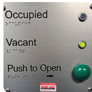
Level 1 accessible toilet entry button
