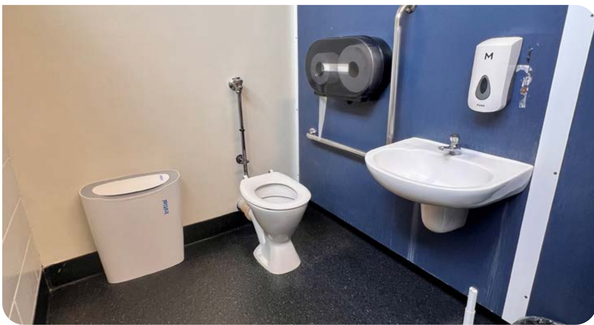
Accessible toilet located on ground floor
